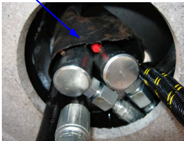
Photo taken looking up from the crane box. Image is for illustrative purposes only, actual crane installation may vary. The pressure, return, and rotation hoses are wrapped in the hose sleeve.
